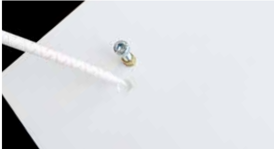
Fill the hole to half its depth with KRION™ adhesive.
